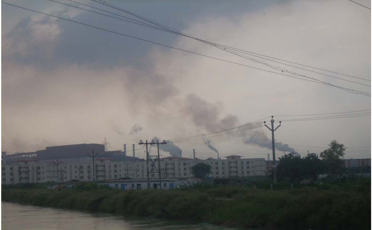
Industrial Pollution Toranagallu, Karnataka - 1
