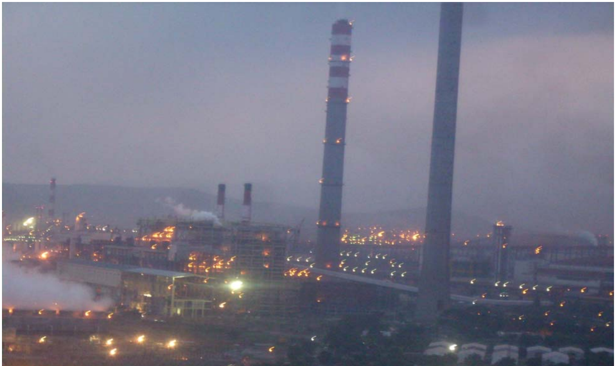
Industrial Pollution Toranagallu, Karnataka – 2
