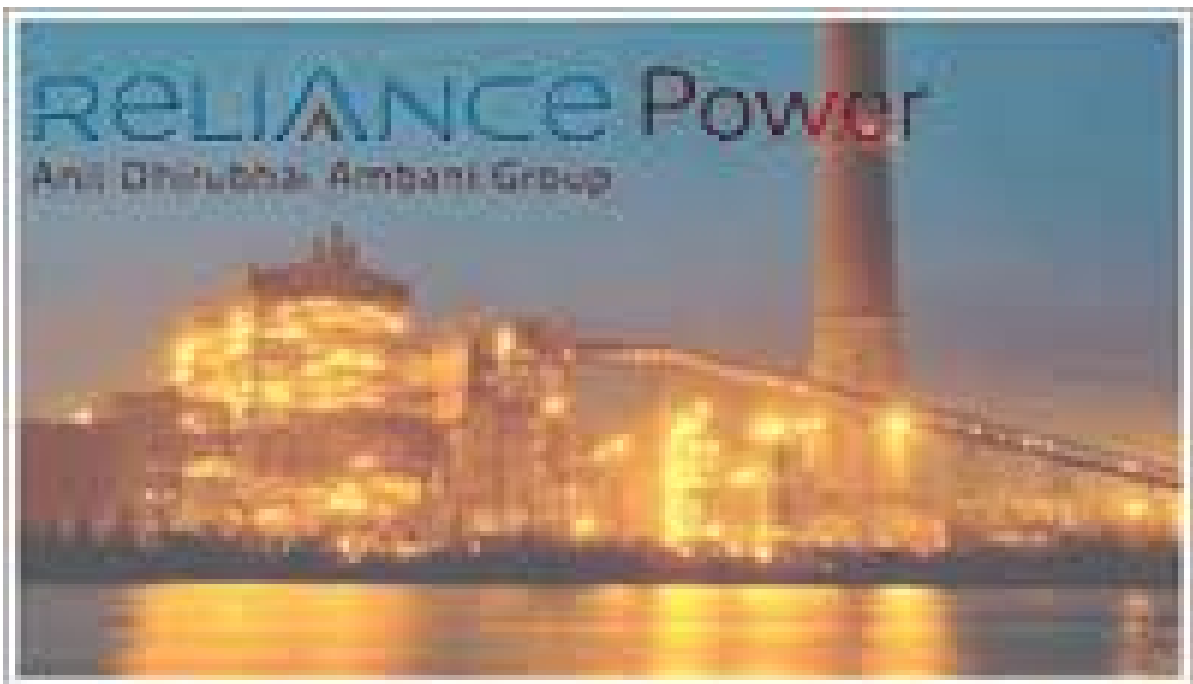
Reliance Power Plant at Sasan
