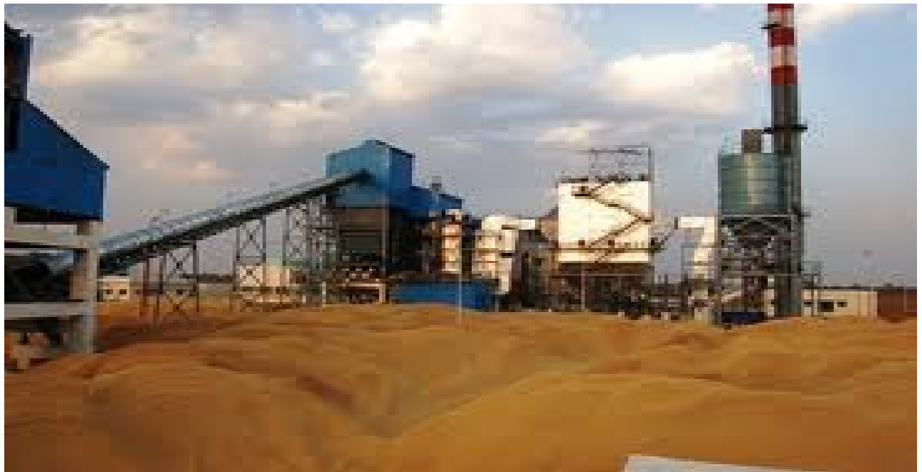
10 MW Biomass Power Project, Gadchiroli, Maharashtra
