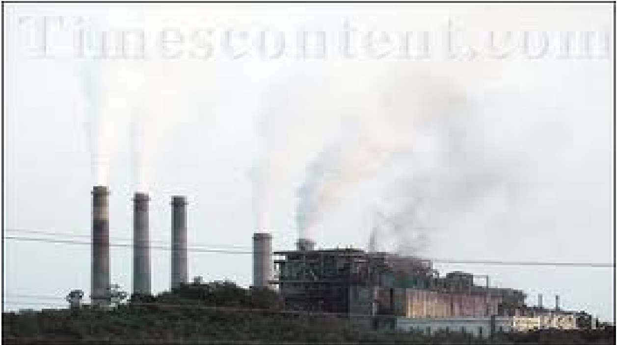
Koradi Thermal Power Plant
