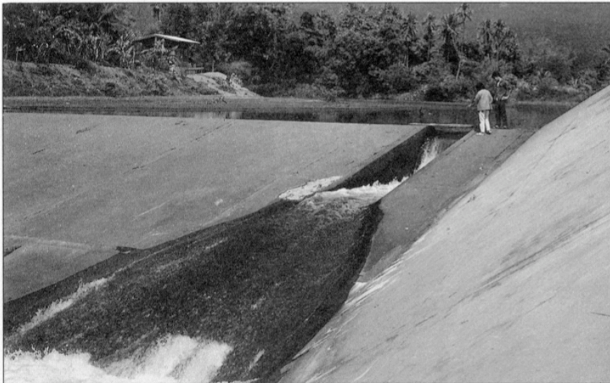
A modern concrete muang faai dam. The concrete dams rapidly clog up with silt and debris, requiring special machinery to clean them out. The amount of labour and finance needed to maintain an "improved" muang faai system is often prohibitive and may cause the system to fall into disuse. (Photo: Chatchawan Tongdeert)
