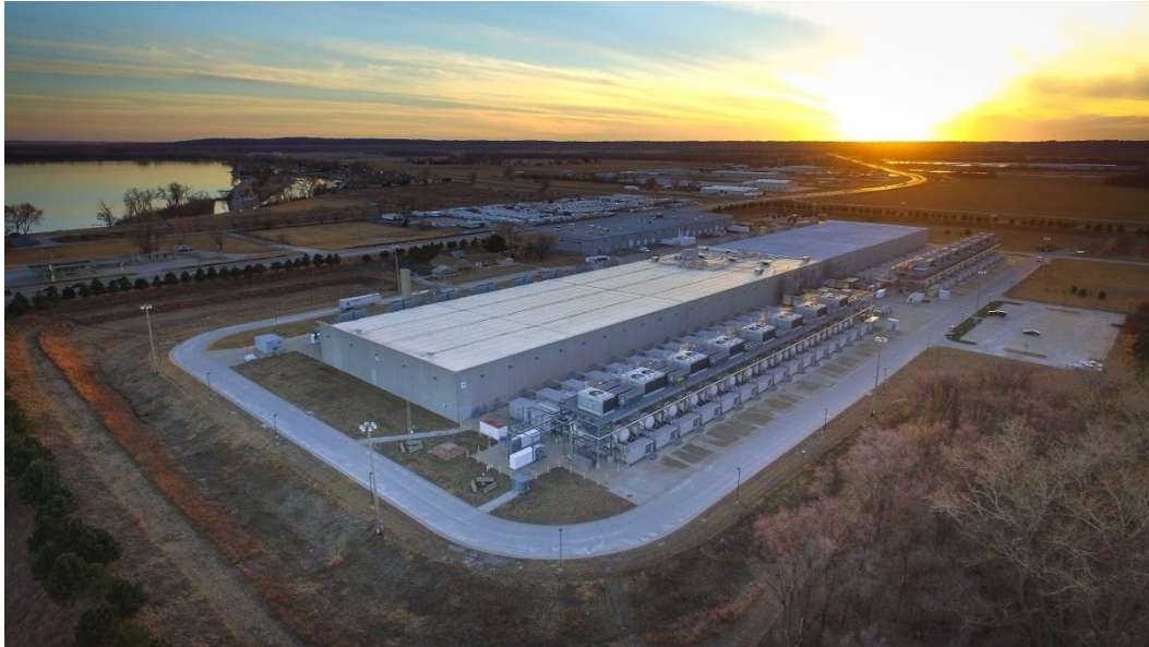
Google's data centre in Council Bluffs, Iowa (Wikimedia)
