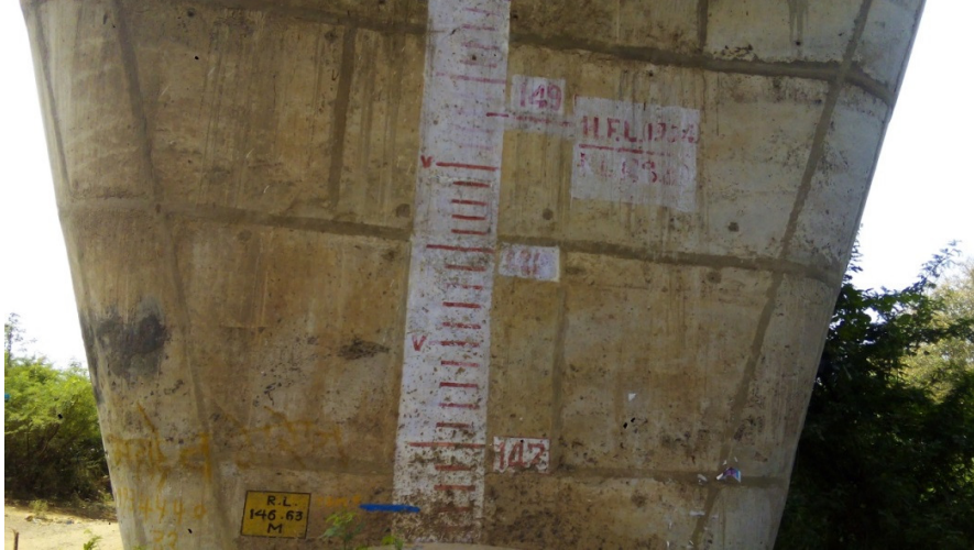
High Flood Back Water Levels marked on a pillar of the Mumbai-Agra highway, shows much higher levels than newly marked NBWL (picture above).
