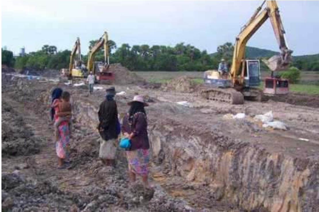
Construction underway on the pipeline to the electricity plant.
