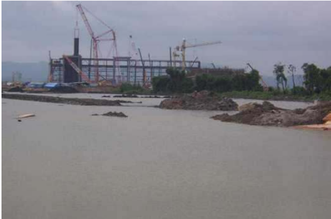
The site of EGAT's new power plant in Chana district.
