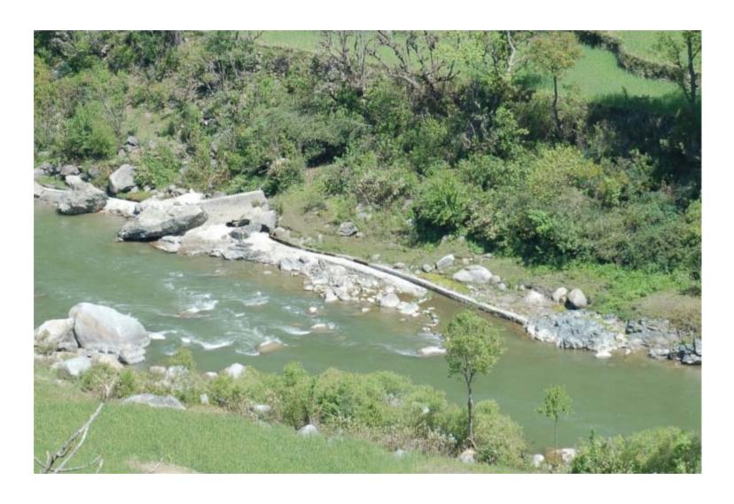
... Using porous rock dams to divert water gently into larger channels while letting silt through . . .
